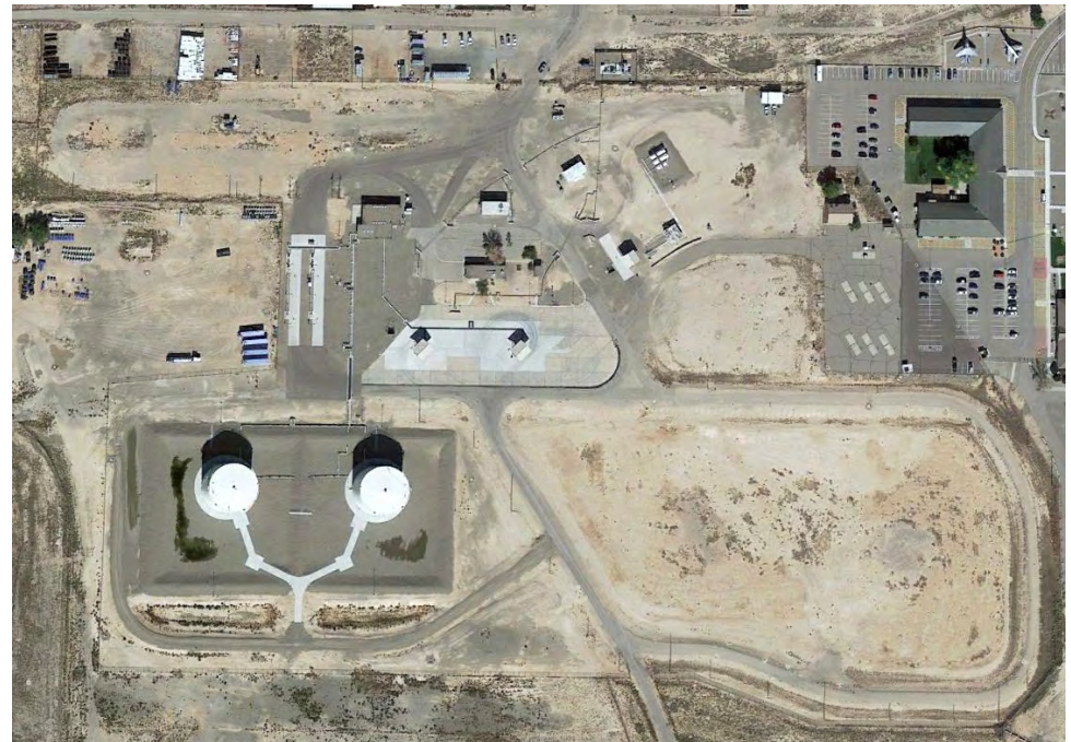
4) November 2015, current infrastructure. Former jet fuel aboveground storage tanks have been removed.
