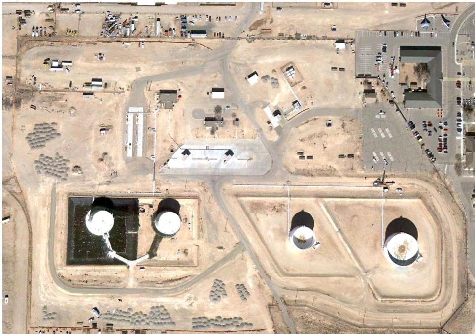
3) February 2011, construction of new infrastructure including new offloading pad and new jet fuel aboveground storage tanks.
